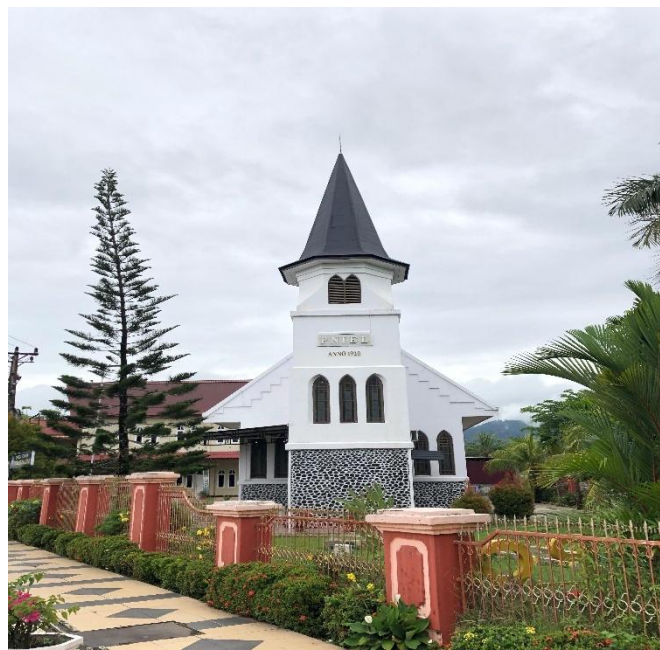
Figure 4. 33. The Church view on front
