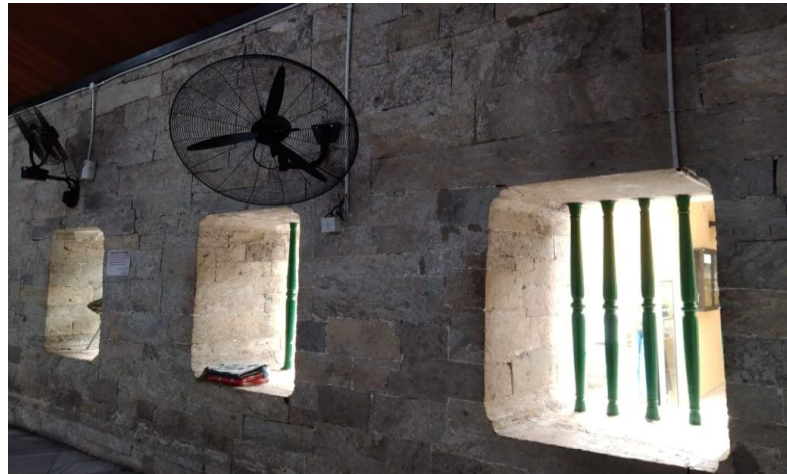
Figure 4. 28. Windows with new wooden posts installed.
