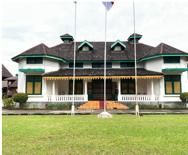
Figure 4. 1. Building seen from the front
