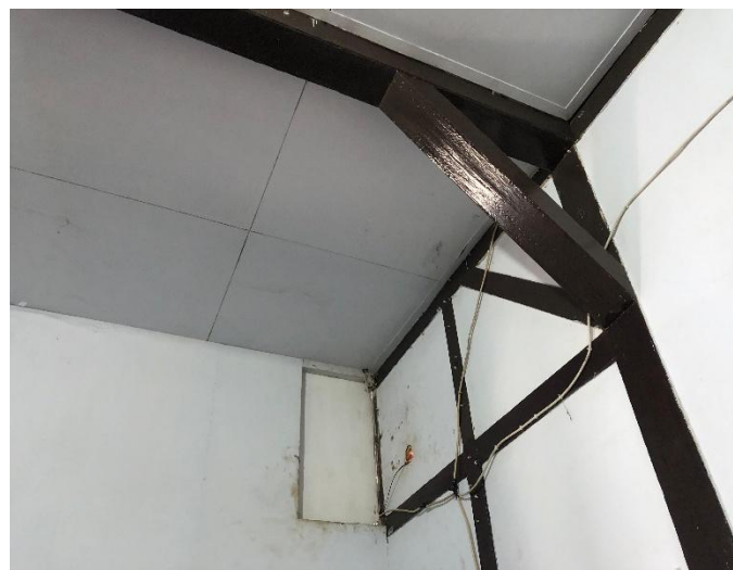
Figure 4. 89. Poles inside the building
