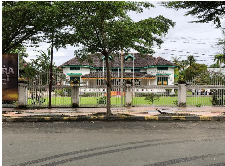
Figure 4. 3 west front of the building from outside the yard
