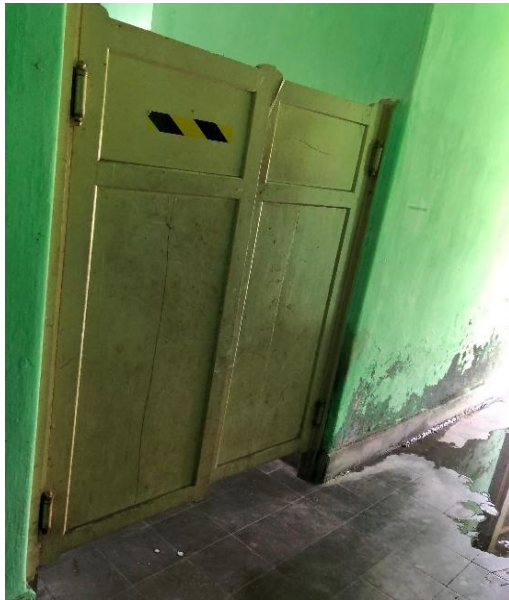
Figure 4. 75. Wood gate inside the mess
