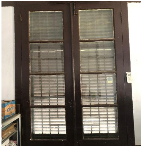
Figure 4. 91. Window inside the building
