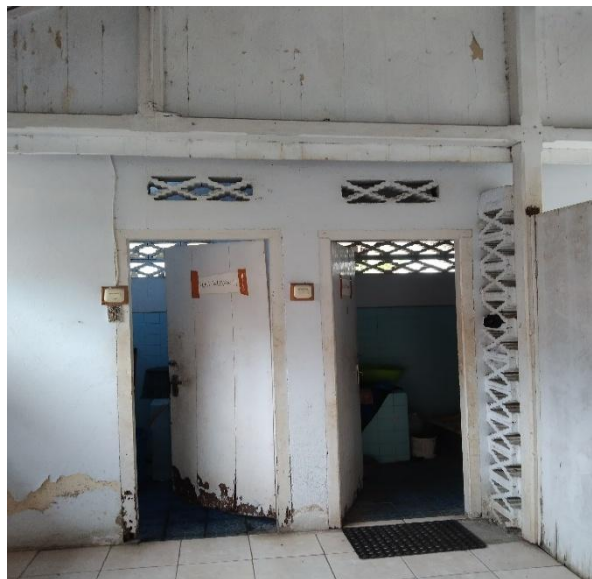
Figure 4. 61. Bathrooms of the building
