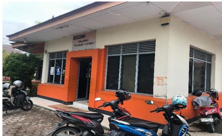
Figure 4. 46. front view of the building
