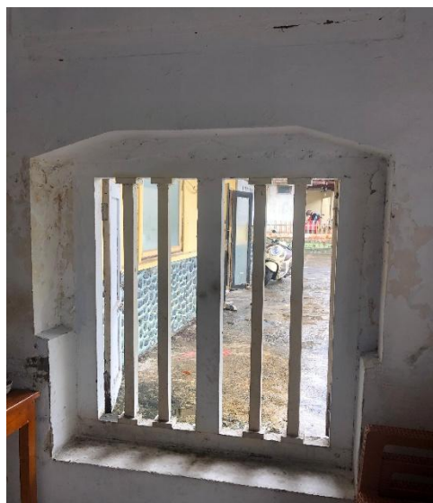
Figure 4. 83. Window in the building
