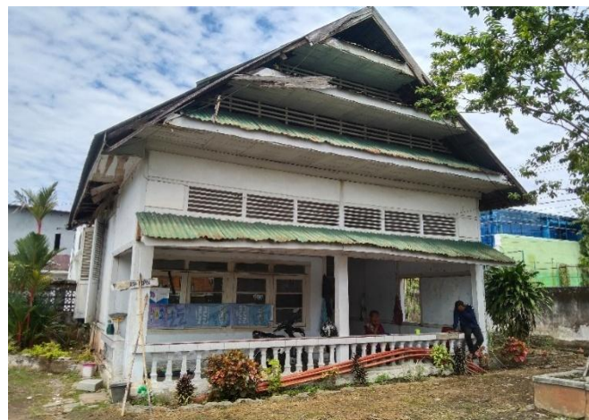
Figure 4. 62. Building beside the building
