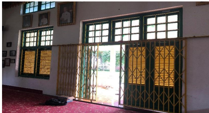
Figure 4. 17. Seen from inside the main door which has been fitted with iron
