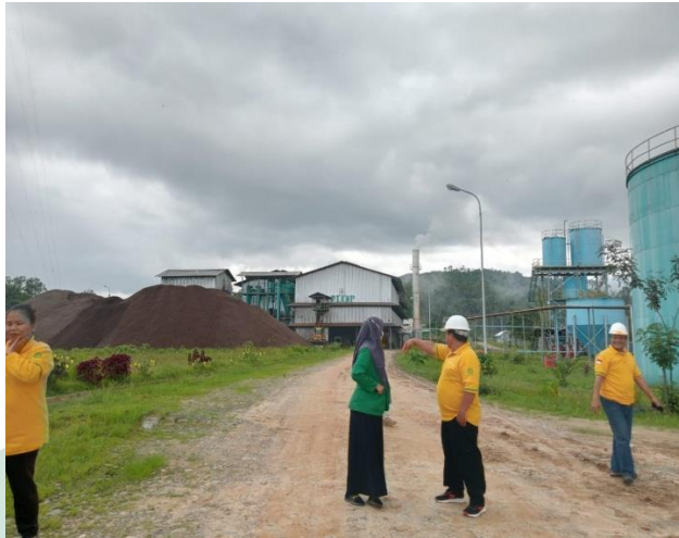
Area Pabrik PT. Kasmar Matano Persada
